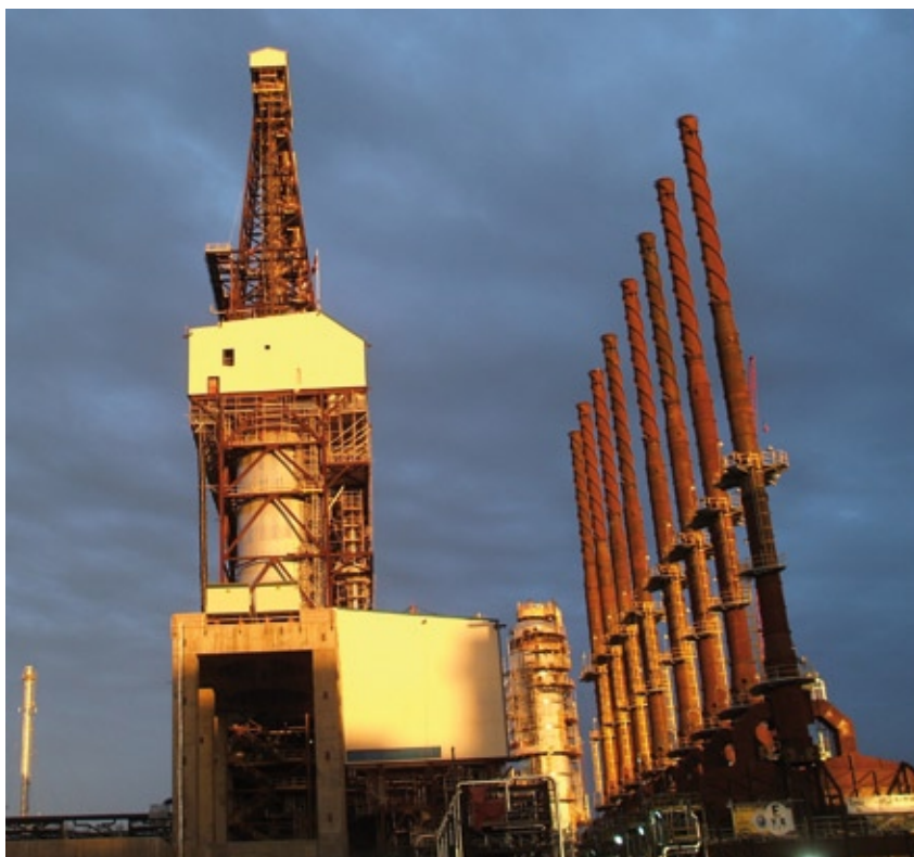
Coker Structure & Delayed Coker Unit Heaters
